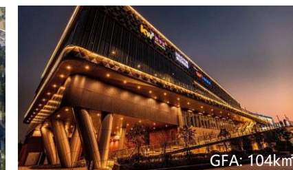
| Jingjiang InCity occupancy rate has stayed at 95% since its inauguration
